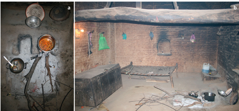
Figure 1. Built hearth structure ( chulha ) in Rajasthan, India, 2017: (a) top view and (b) side view. This chulha has two U-shaped chambers to accommodate two cooking fires simultaneously, although only one fire is burning. In each chamber and in the front, the chulha is slightly deeper than floor level to provide more space for the firewood. The rear of the chulha is a useful space for storing kitchen equipment, such as the bowls and clay griddle seen here. The house has carbon stains on the interior walls, floor, wooden beams, and furniture from the soot and smoke. Photo by M. Beck.
